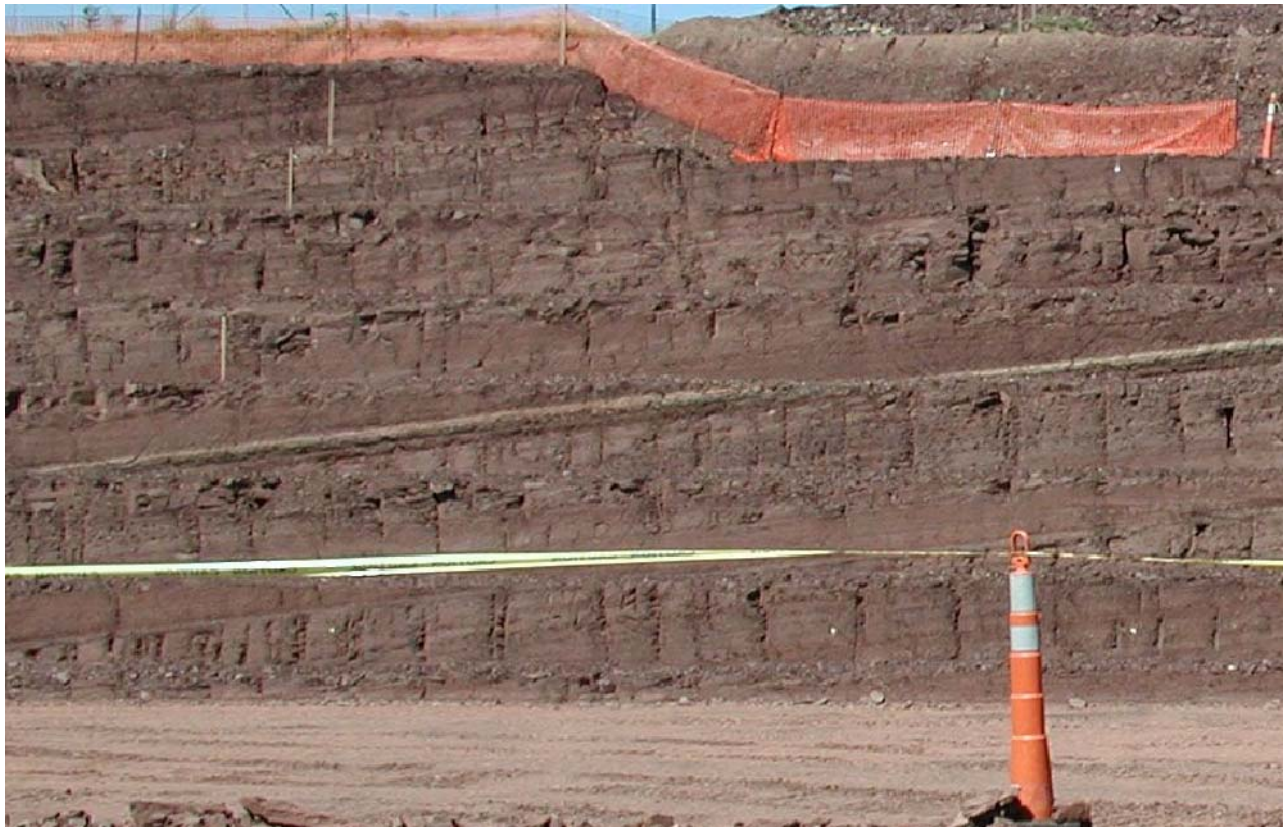
Figure F15. Extension fractures in mudstone and siltstone of the Passaic Formation (Brunswick Middle Red zone) exposed in vertical face cuts during excavation of a commercial pipeline, Somerset County. Plastic netting on the upper benches is about 4 feet in height. Note the difference in thickness between bedding and fractured layers and how fracture density and dimensions differ. Photograph courtesy of Don Monteverde, NJGS.
